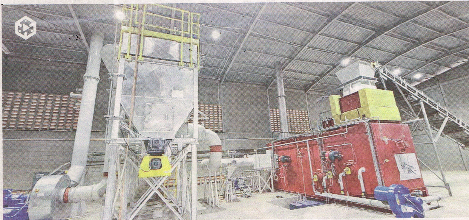
One of the 16 regional incinerator hubs the Government is constructing in Lira to handle hazardous medical waste from Lango sub-region. (Scan photo using Vision Digital Experience to watch video)
