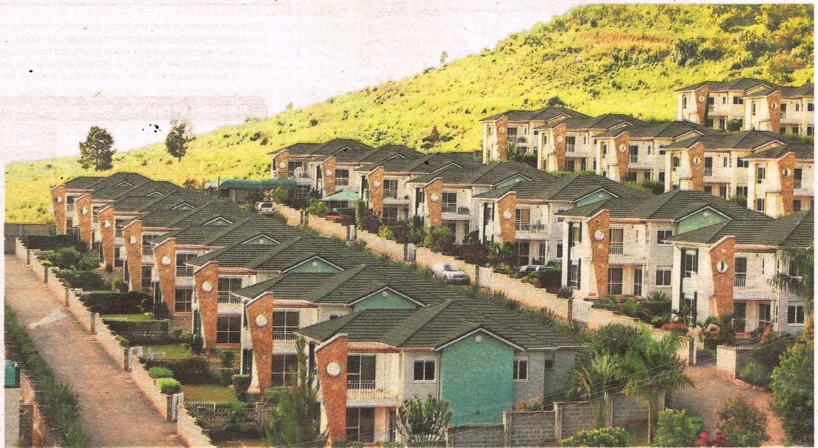
Condominiums in Lubowa, a Kampala suburb. MPI is often embedded in loans to protect mortgage portfolios from large-scale defaults. PHOTO/FILE
